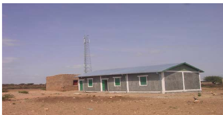
School constructed in Somali region
