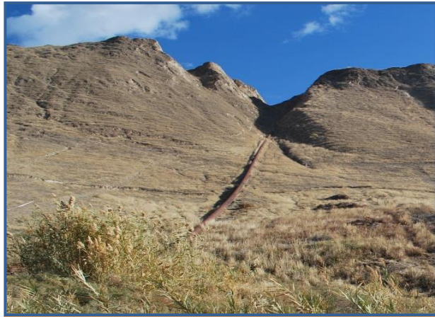
Water supply projects along “Panj” river
