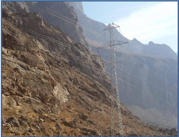
Construction of transmission/communication lines Darvoz, Vanj and Khovaling districts.
