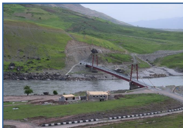
Construction of transboundary bridges “Shoun”, “Vanj” and “Kokul”
