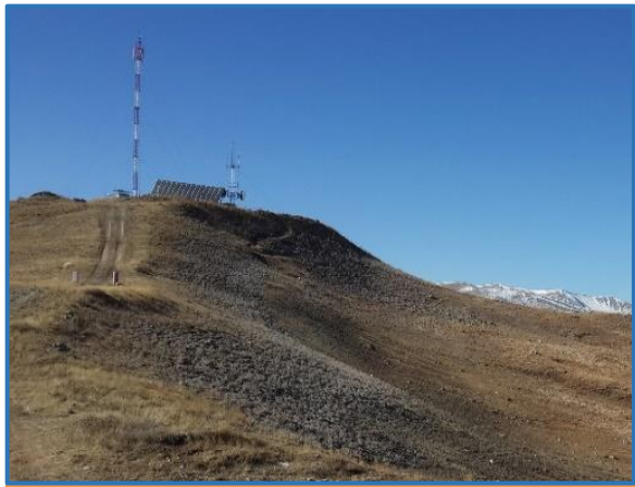
Installation of communication network in Saghirdasht of Darvoz district.
