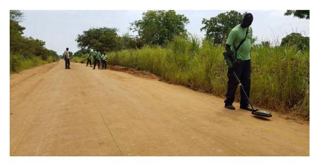
The majority of the suspected mined roads in South Sudan are devoid of vegetation and believed to only be contaminated with anti-vehicle mines. As such clearance is done using a combination of dual sensor detectors and mine detection dogs in a deployment style that achieves 1 km of road clearance per day  $(8,000\text{m}^2/\text{day})$ . Therefore, road tasks are disaggregated from other demining tasks, as the speed of clearance is so different.
