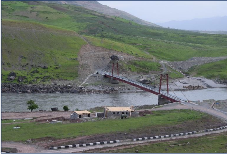
Construction of transboundary bridges “Shoun”, “Vanj” and “Kokul”
