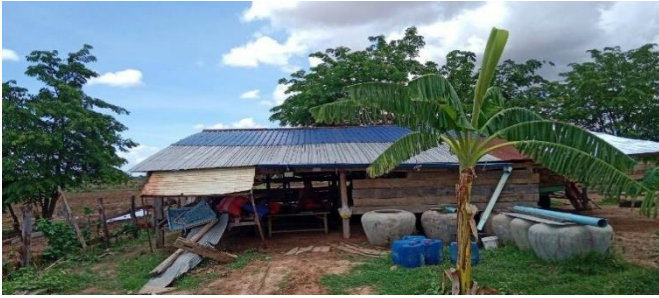
Figure 4: This house's ground was cleared to ensure safety of the residents
