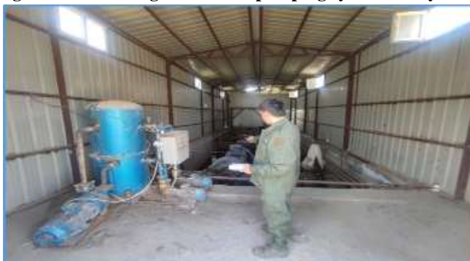
Pumping units of the integrated water pumping system in Jayhun district
