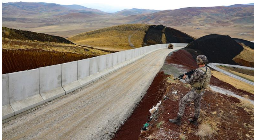
Photo-1: Modular concrete walls and patrol roads of IBM System
