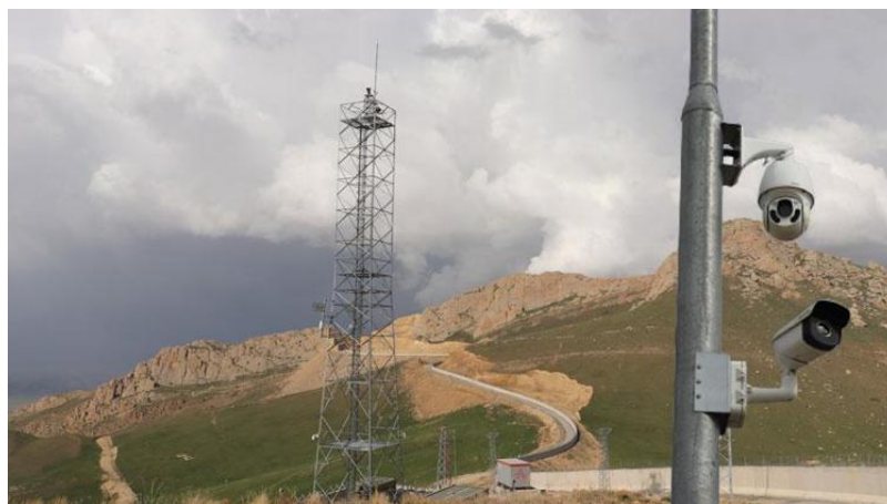
Photo-2: Modular concrete walls, patrol road and IT aspects of IBM System
